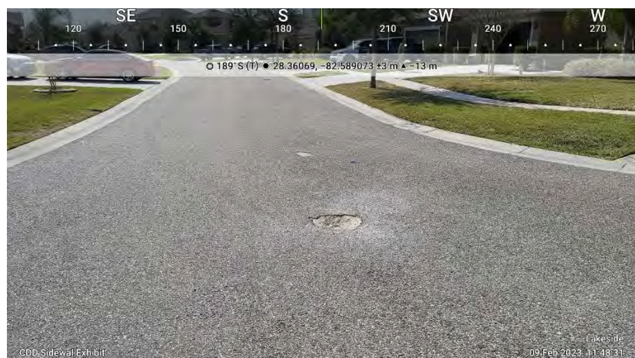
Figure 1 Existing Pothole
